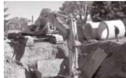
As part of "Operation Overflow," sanitary sewer pipes were placed over 30 feet deep in some areas under Appleton and Skye Drives.
