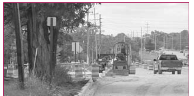
Road construction in Farmington Hills.
