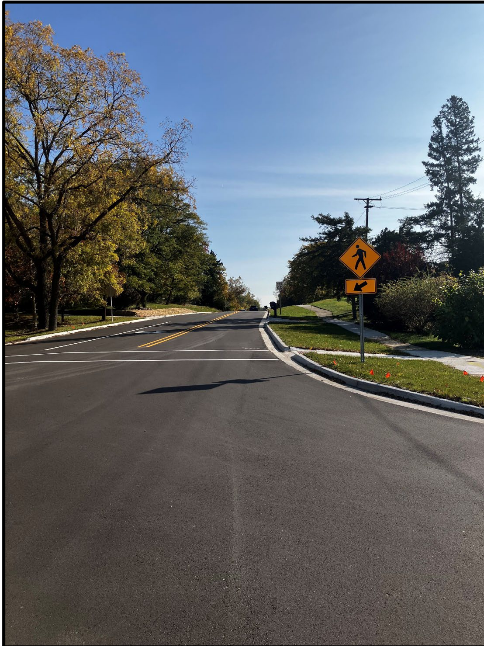
Eleven Mile Road repaving at Power Road
