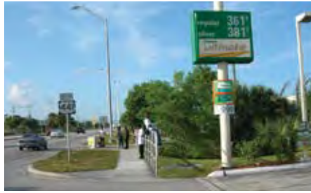
Photos of existing conditions on State Road 7 show an automobile-dominated corridor with few amenities for transit riders. (STATE ROAD 7 COLLABORATIVE)
