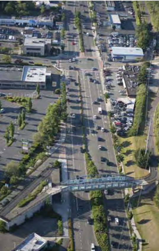
Improvements along the Aurora Corridor have included a new pedestrian bridge, landscaped medians, and upgrades to utility infrastructure. (HDR ENGINEERING INC.)
