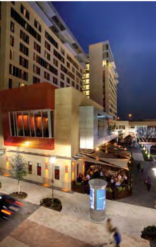
CityCentre features carefully crafted design elements and landscaping. (CITYCENTRE)
