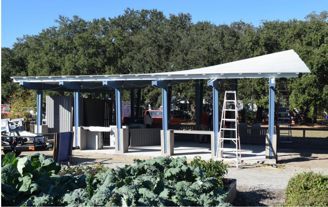
Completed Medway Park, Charleston North Carolina
