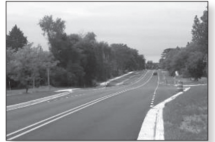
Ten Mile Road after paving.
