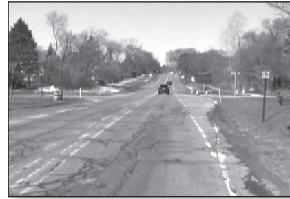
Ten Mile Road before paving.
