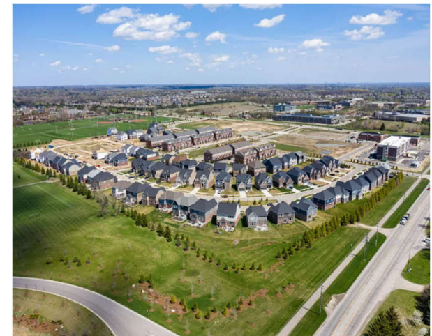
Village at Northville Northville, Michigan 102 Single Family Homes, 64 Townhomes, 283 Multi Family Units, 88,000 SF Commercial
