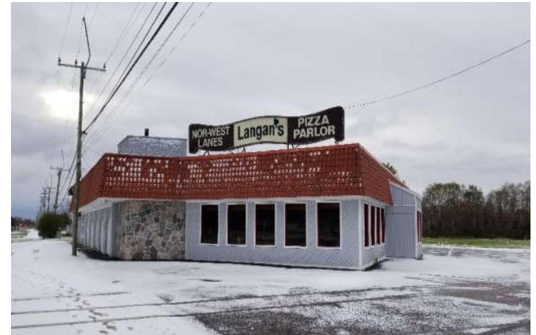
Current View of Nor-West Lanes
