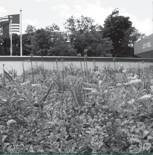
The City Hall green roof filters stormwater and reduces heating and cooling costs.
